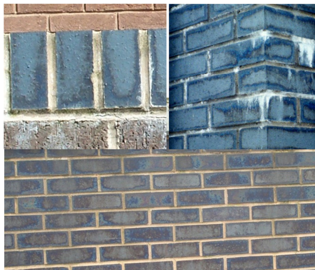
Iridescent appearance caused by light diffraction through fine cementitious material that has leached from mortar.
