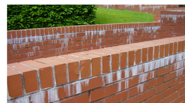
Lime stains emanating from mortar. No damp proof membrane has been incorporated under the brick on edge capping.
